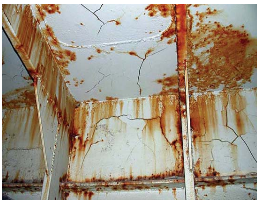
Figure 1. Marine coating degradation showing cracks and rust in water ballast tanks
